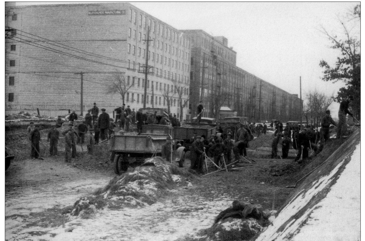
West Allis Street Construction
