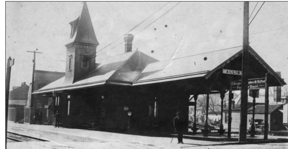
Chicago, Milwaukee and St. Paul Rail Road Depot
